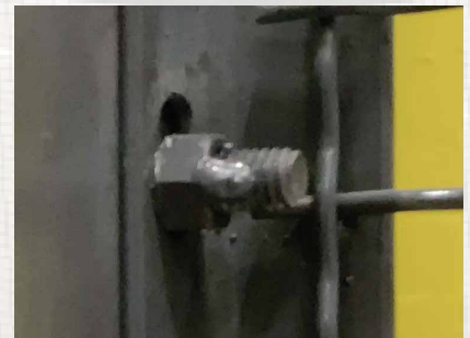
Tamper-proof hardware on inside of cage.
