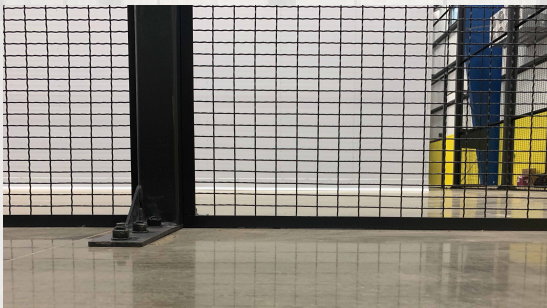
Cage panels mount flush to floor.
